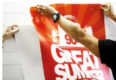
3. Remove the air between the film and the applied surface to assure strong adhesion. You can use the cardboard backer for this.
